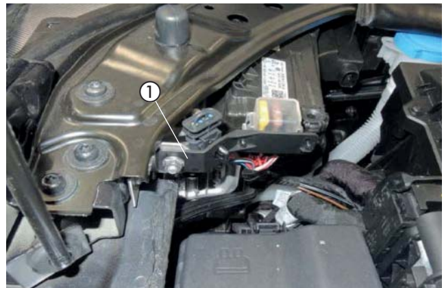
Fig. 44 ① Fuse block holder mounted to 90° angle bracket
