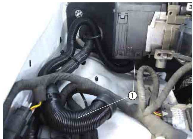
Fig. 24 ① Connect and lay combustion air pipe
